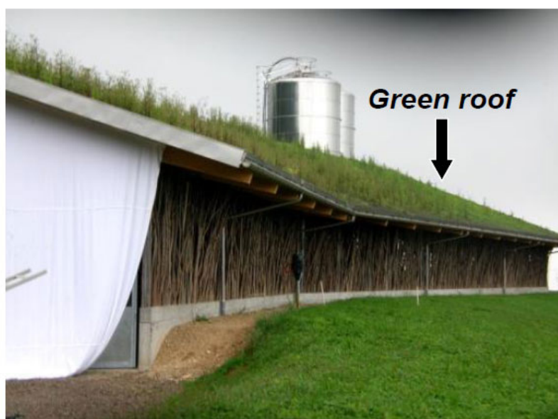
Fig. (6). Green roof used in dairy cattle housing [26].
